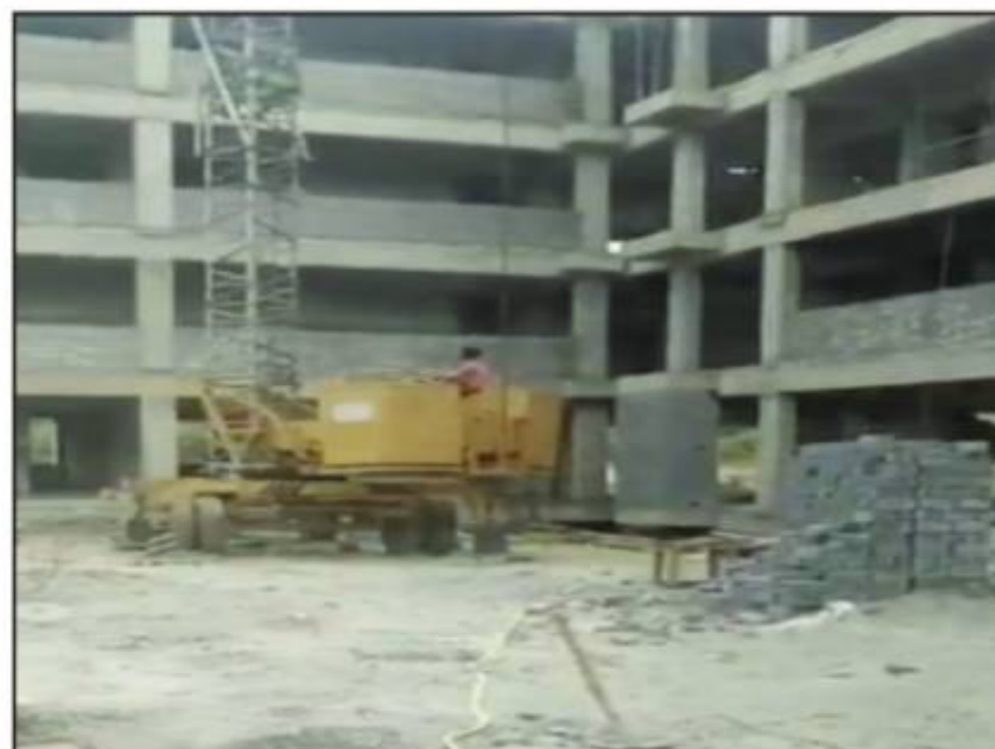
School Building at durga park, dwarka
