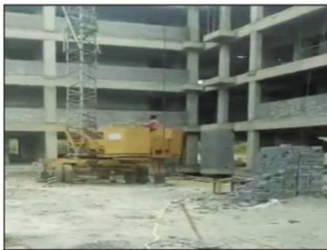
School Building at durga park, dwarka
